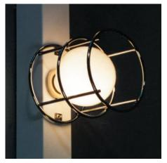
The wire guard conforms to NEC requirements for dressing rooms.
